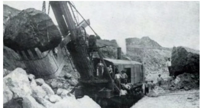
Marion Steam Shovel Model 90, pictured in 1908 at work on the Panama Canal. Image credit: Wikipedia.
