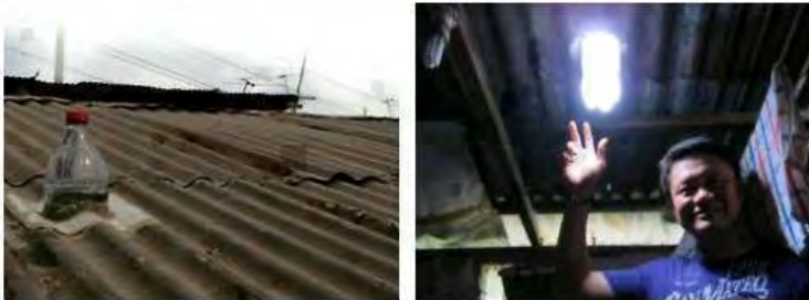
To the left, this non-electric "bulb" was made in the Philippines. Water and bleach were added to a plastic bottle and the bottle was fitted onto the roof. It absorbs and reflects the sunlight and is equal to 55 watts.
